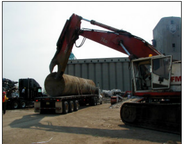
Inspection: Tanks are cut open and checked prior to unloading
